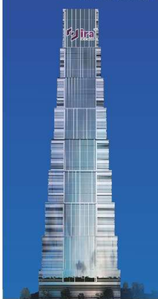
GATEWAY TOWERS, PUPPALAGUDA
