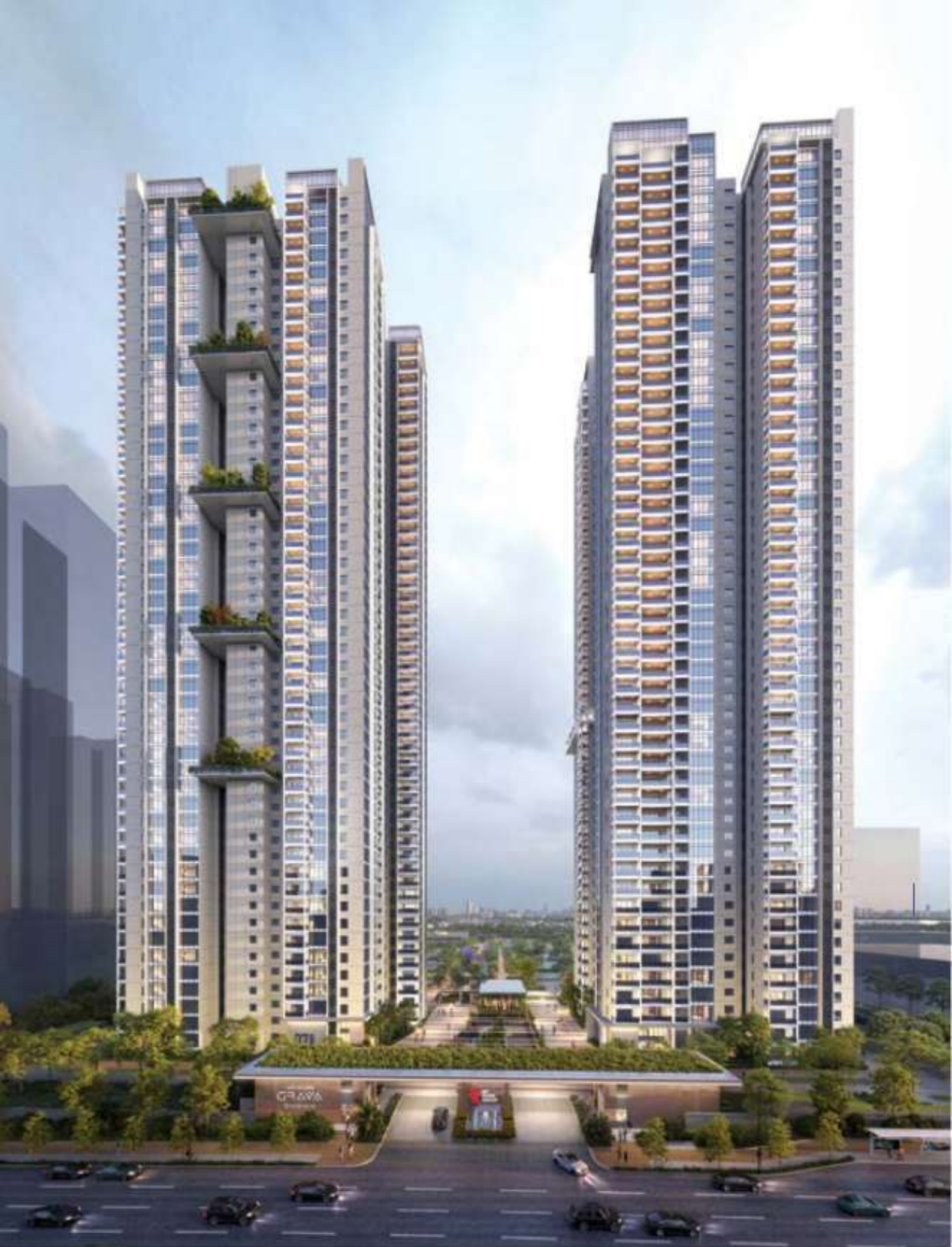
Towers, North View
