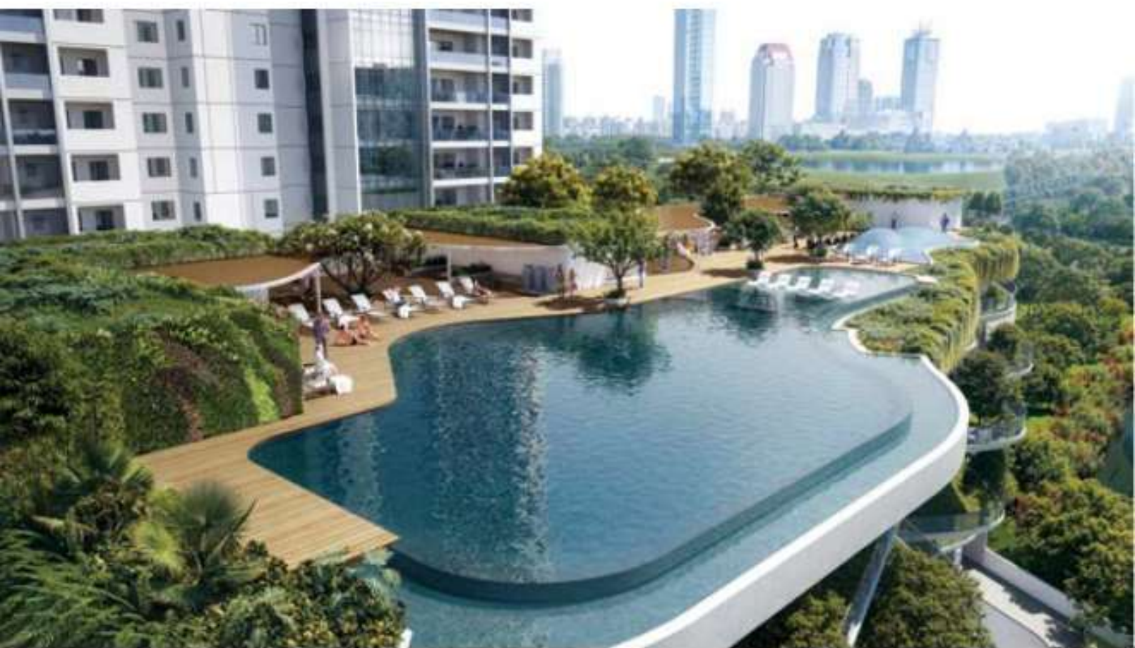
Temperature Control Swimming pool on Clubhouse Terrace
