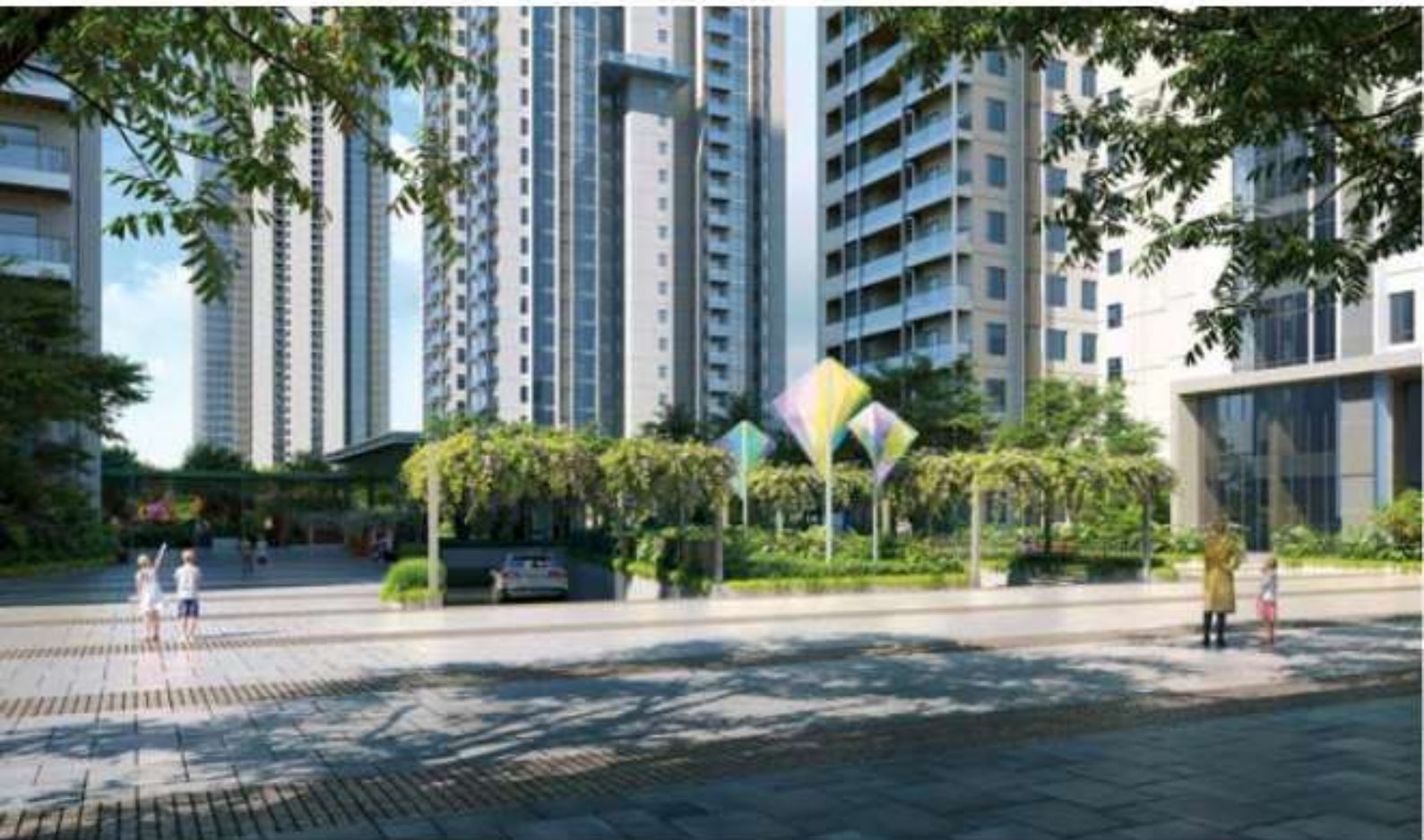
Entry Ramp To Basement
