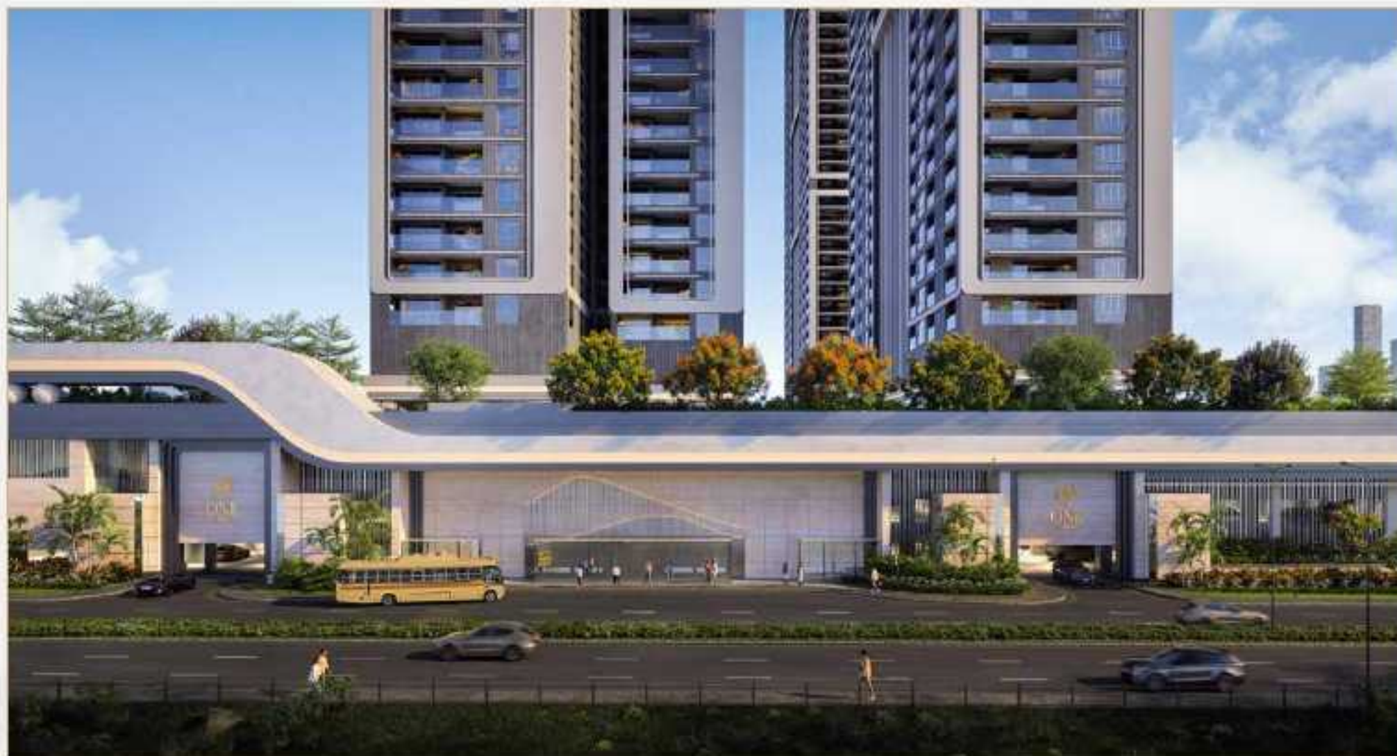
DUAL ENTRY/EXIT GATES
